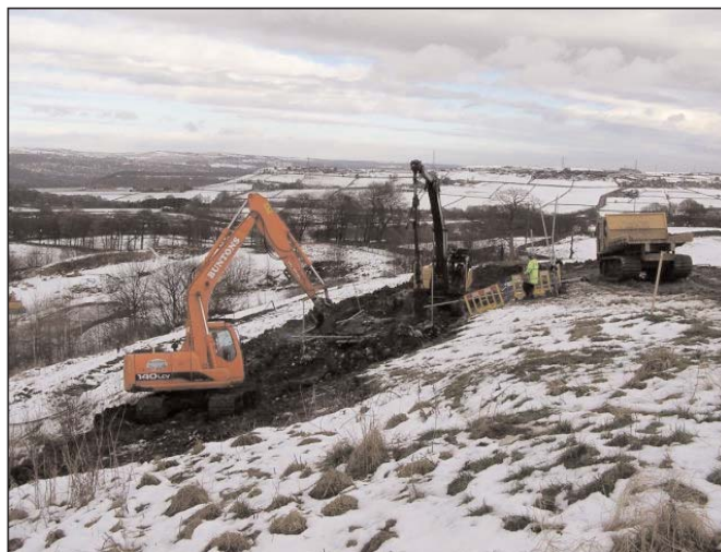
Bradford Council will now carry out major works at Manywells
